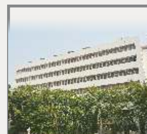
Central Library Block-C
