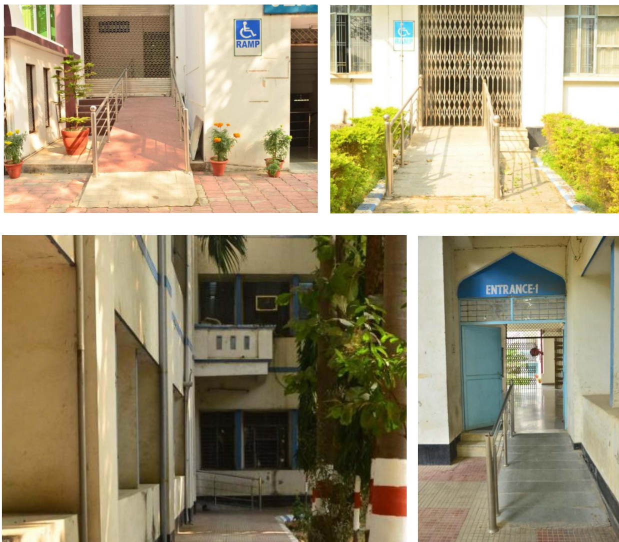
FIGURE 29: Provision of Ramp with proper handrails at every entry/exit of the Department.
