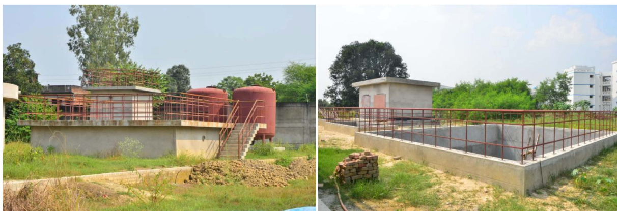
FIGURE 10: Sewage Treatment Plant (under construction)
